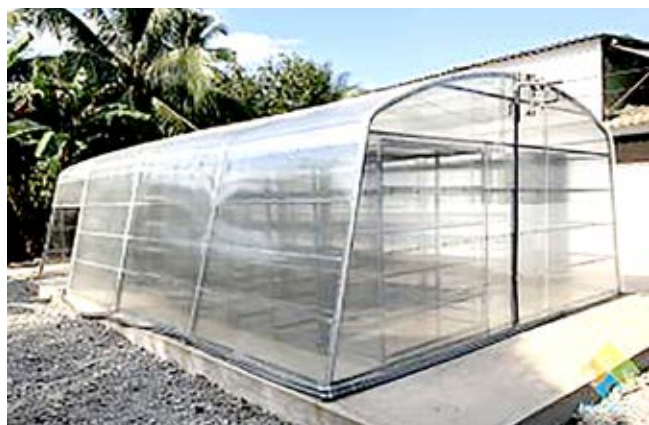
The solar drier is a simple greenhouse-like structure that uses solar energy to dry farm produce which is later packed and stored for future use or sale.
