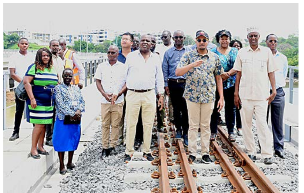
PS Mohamed Daghar leads a delegation of senior government officials in inspecting the MGR line at the Makupa causeway in Mombasa County.
