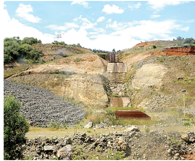
An abandoned section of Itare Dam site, in Kuresoi North, Nakuru County.
