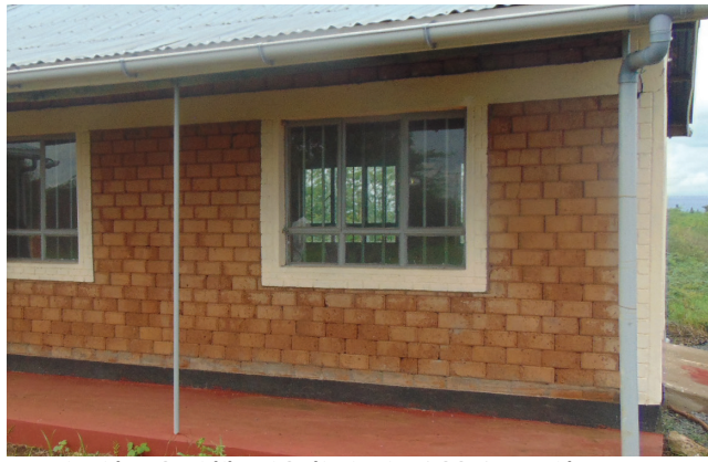
Interlocking Stabilized Soil Blocks (ISSB) used in construction of government offices in Taveta
