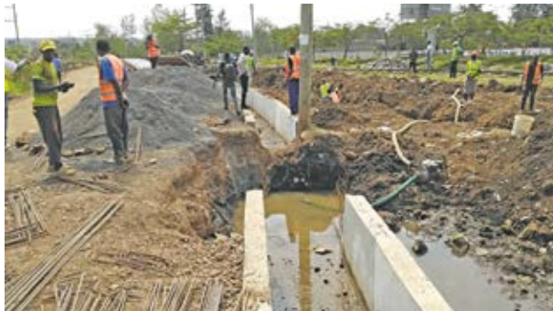
A section of Auji-Pundo road in Bandani informal settlement under construction
