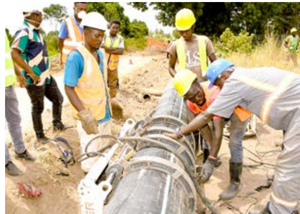
Kwale Water and Sanitation Company Ltd workers installing bulk water pipes in Diani municipality to ease access to clean water and sanitation. PHOTO: HUSSEIN ABDULLAHI
