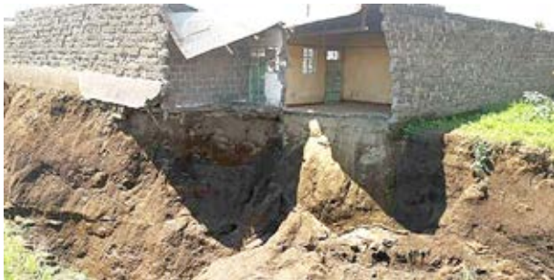
Deserted houses that were destroyed by a sinkhole in Nakuru area.
