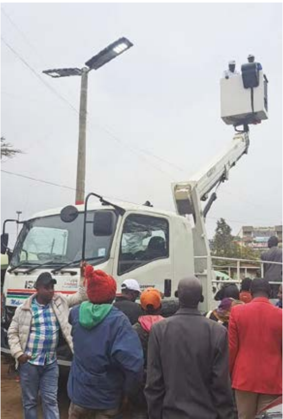
Kiambu’s 23-meter manlift in action, supporting streetlight installation and maintenance for safer public spaces.
