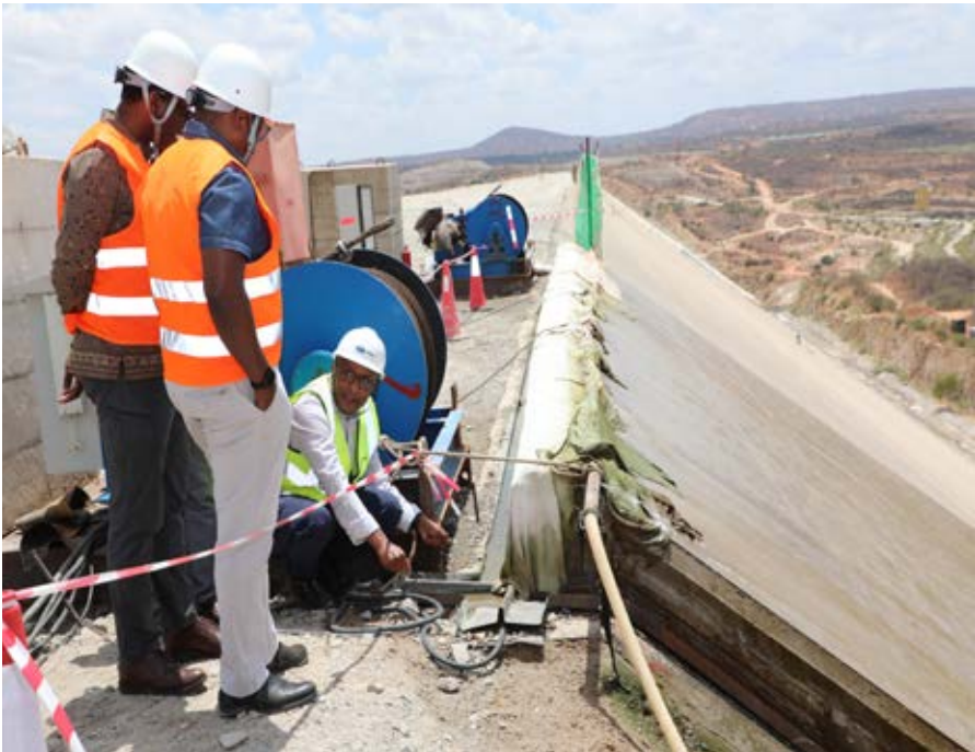
Concrete face slabbing underway at the Thwake Multi-purpose Dam. Phase is scheduled to be complete in the next eight months with the construction of a bridge to connect Kitui and Makueni besides installation of hydro-mechanical equipment and gates.
