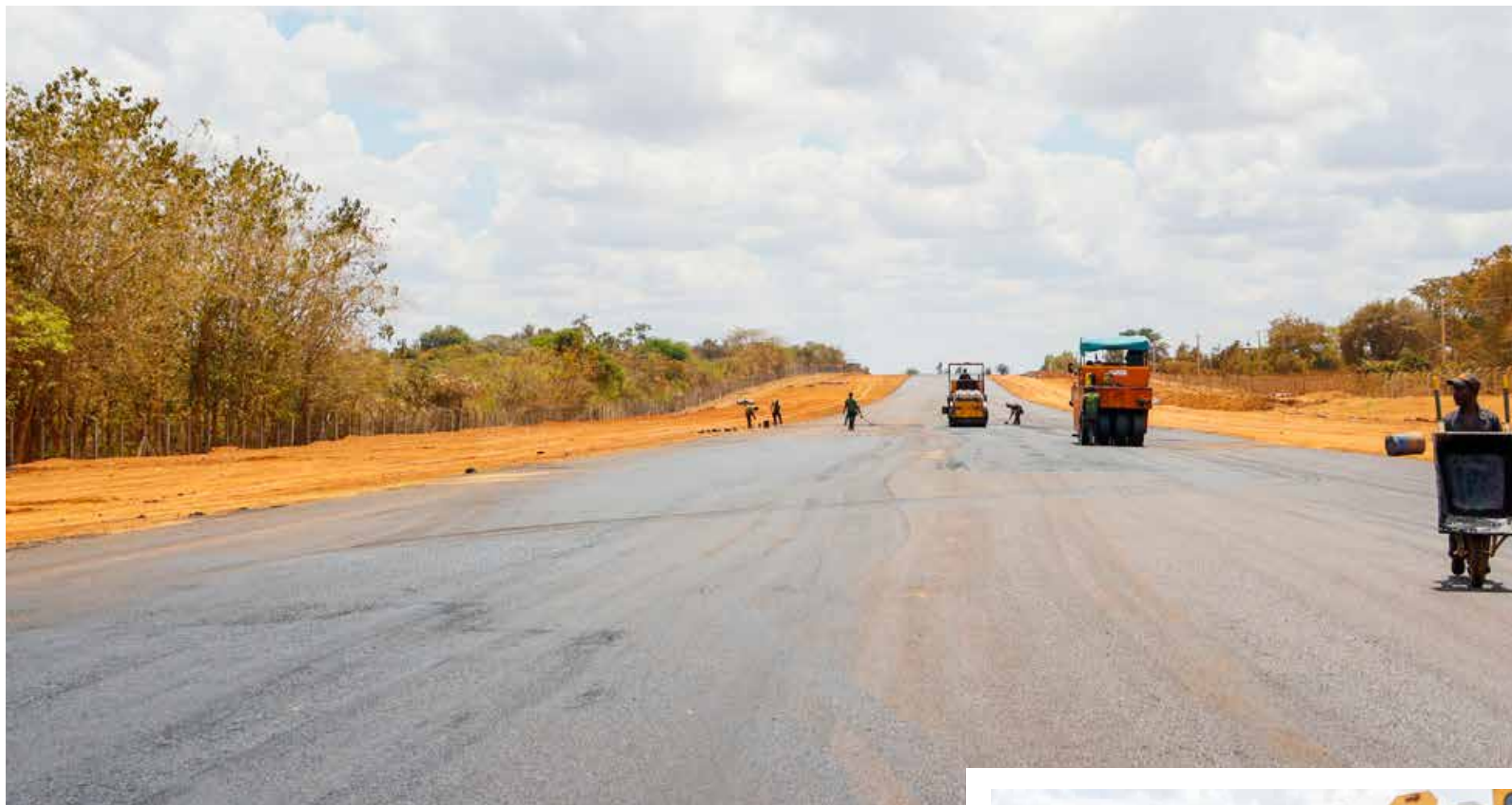
The new Ithookwe Airstrip runway that stretches 950 metres in length and 18 metres in width, a significant expansion from its previous state.
